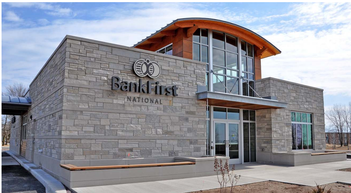
Bank First National's newest office located at 1703 Lake Street, Two Rivers, Wisconsin.
