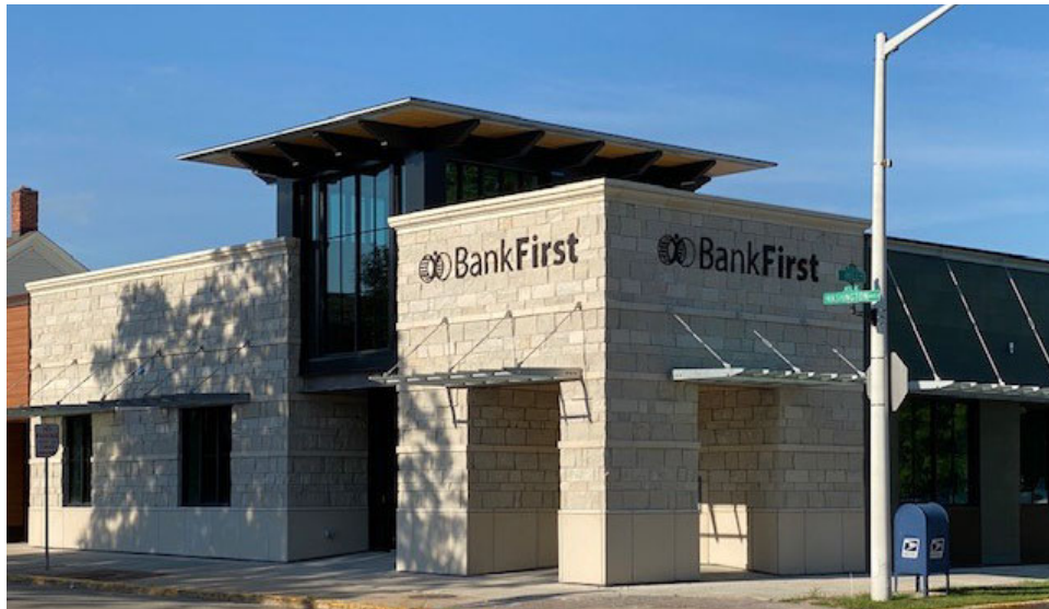
Photo of Bank First's newly renovated office located at W61 N529 Washington Avenue in Cedarburg. Construction of the facility began in October of 2019 and the official reopening date is set for July 27, 2020.
